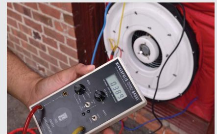
Deep Energy Retrofit
