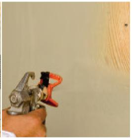
3. Apply Sto EmeraldCoat® onto the entire wall surface. Sto EmeraldCoat® can be used beneath various claddings.
